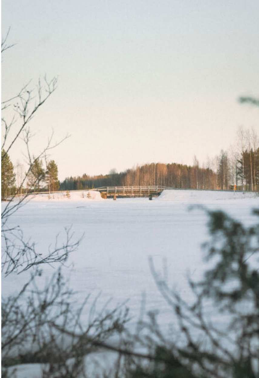
Bridge In Spring Weather Oskari Pulkkinen Finland
