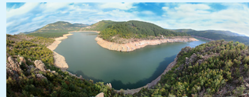
Arda Kardzhali Dam Rope Bridge
